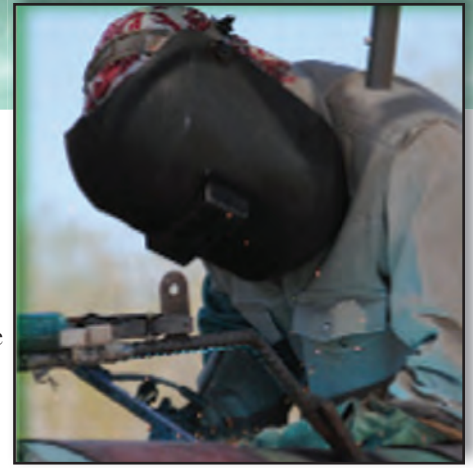
A welder connects pipe on a natural gas pipeline
