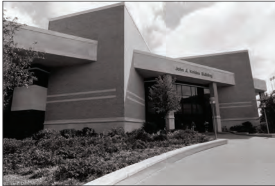
The Koldus building houses the Borrow a Bike Program
